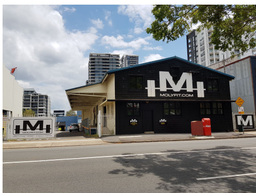
Entrance at 32 Cribb St.
